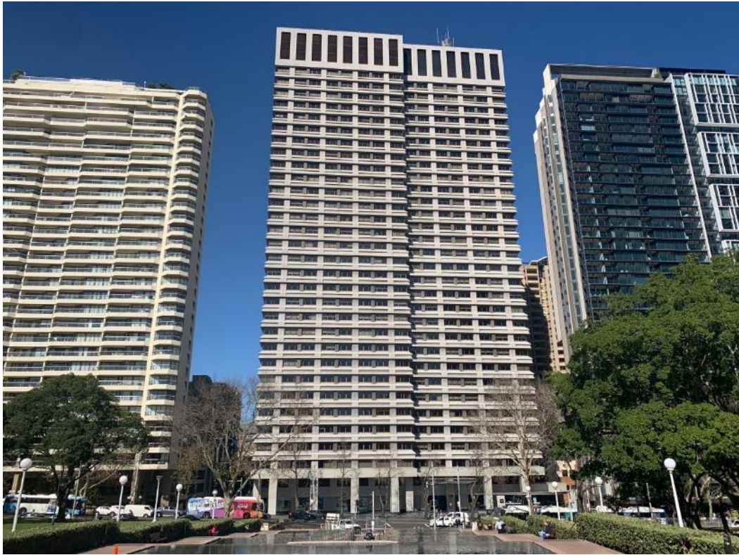
Figure 3: Site and neighbouring buildings on Liverpool Street, viewed from Anzac War Memorial
