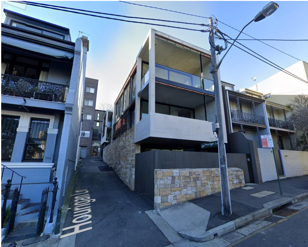
Figure 2. 90 Brougham Street looking east from Brougham Street
