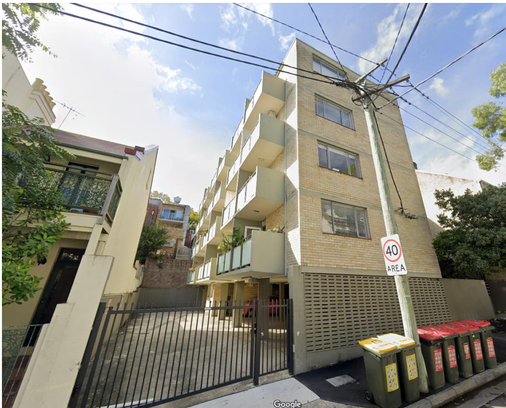
Figure 3. 100-104 Brougham Street looking east from Brougham Street
