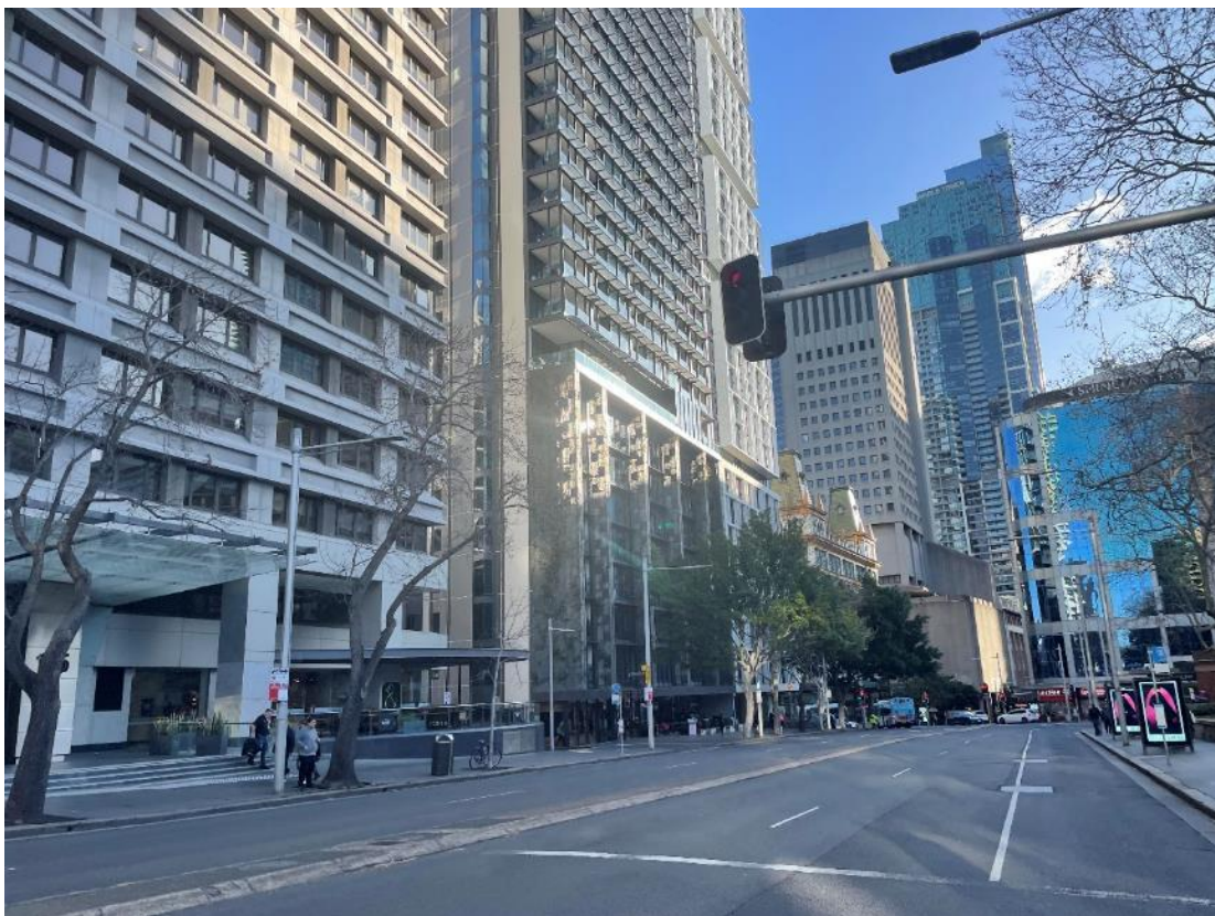
Figure 14: Street level view of The Hyde and the subject site
