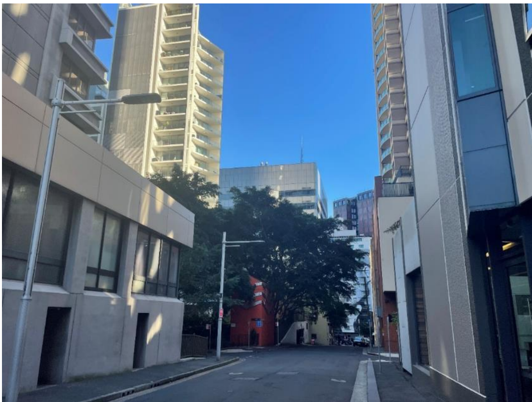
Figure 22: View of buildings along Nithsdale Street, facing south
